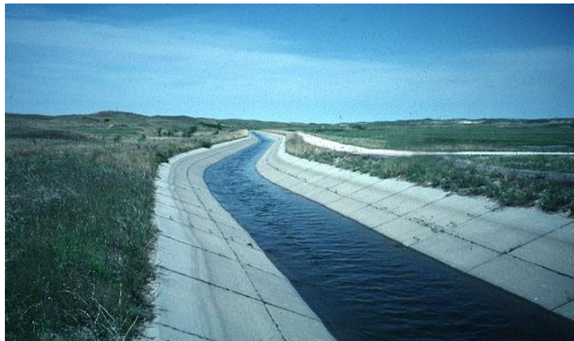
Figure(2): Concrete lining for irrigation canal.
