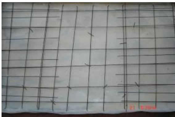
Photo (3) Details of the reinforcement mesh of slab S_3 (case3).
