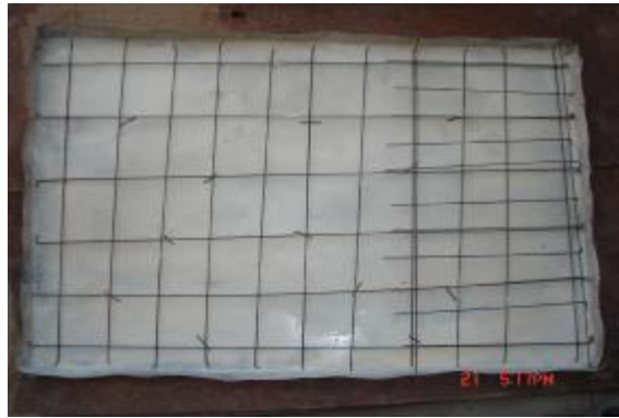
Photo (6) Details of the reinforcement mesh of slab S_7 (case7).
