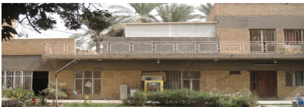
Figure 6: The front of the house is exposed to solar radiation with multiple windows
