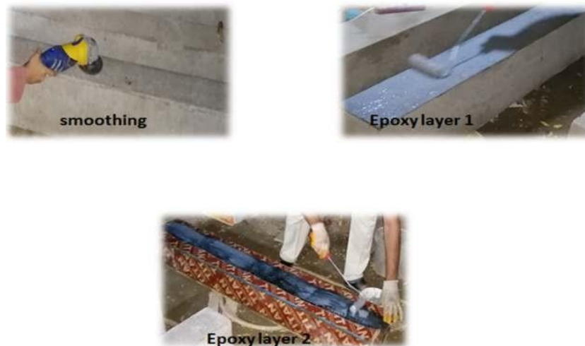
Plate 1. Strengthening of beams with (CFRP)works.
