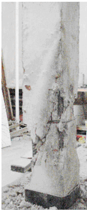
A- Column specimen C 11
