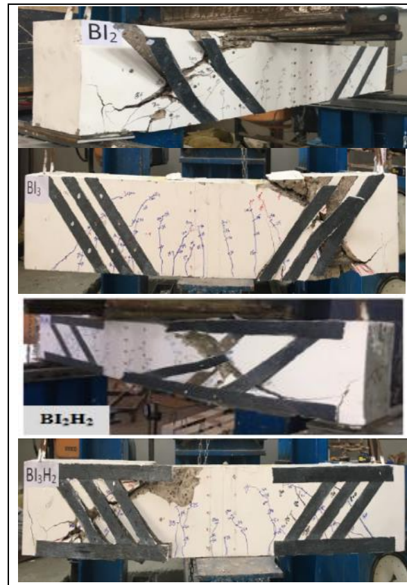
Figures 10. Crack pattern for the beams failed in shear for group (A)
