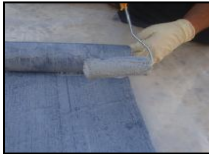
Plate (2) Specimens retrofitting process
