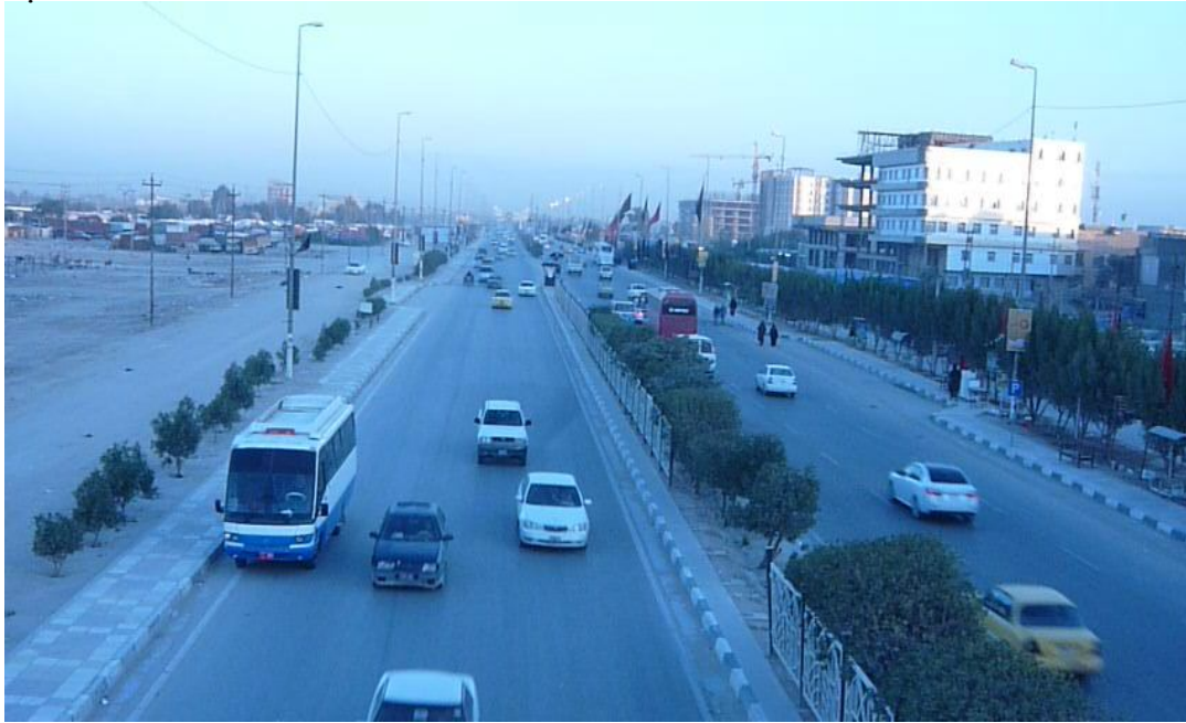
Figure 2 Site1 located on Karbala -Najaf roadway.
