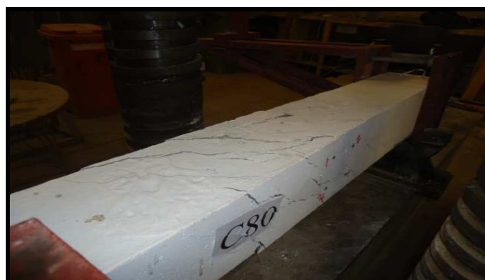
Figure (20), Crack Pattern and Failure Mode of Hollow SCC Beam (C80)
