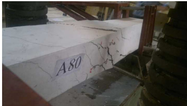
Figure (8), Crack Pattern and Failure Mode of Normal Strength SCC Beam (A80)
