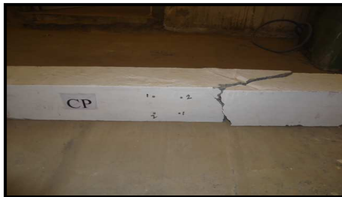
Figure (19), Failure Mode of Hollow Normal Strength SCC Beam (Cp)
