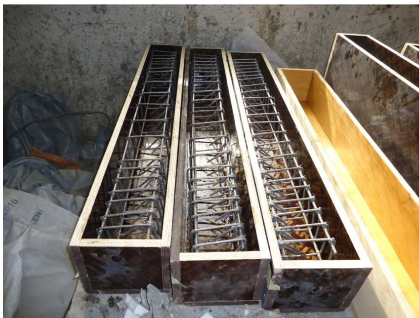
Figure (2). Steel Reinforcement and Wooden Mold
