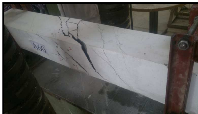
Figure (10), Crack Pattern and Failure Mode of Normal Strength SCC Beam (A60)
