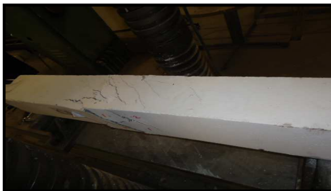
Figure (21), Crack Pattern and Failure Mode of Hollow SCC Beam (C100)
