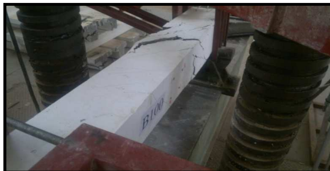
Figure (15), Crack Pattern and Failure Mode of High Strength SCC Beam (B100)
