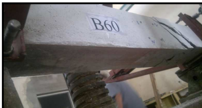
Figure (16), Crack Pattern and Failure Mode of High Strength SCC Beam (B60)
