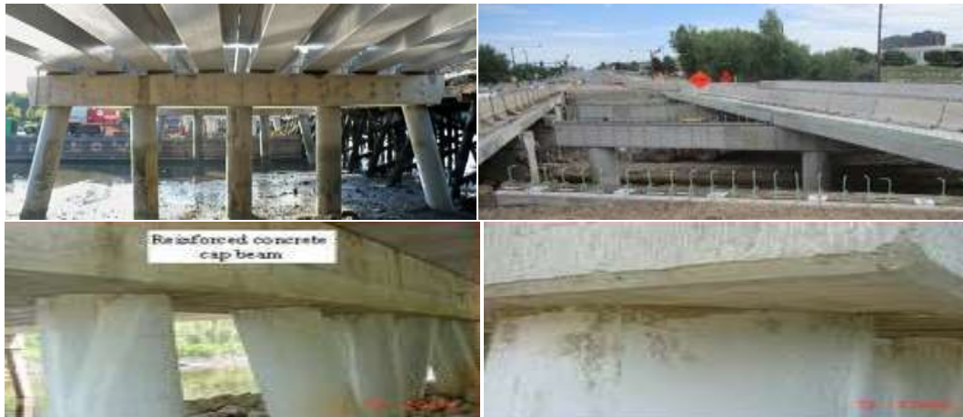
Figure 1: Pile Caps Behave as Continuous Deep Beams
