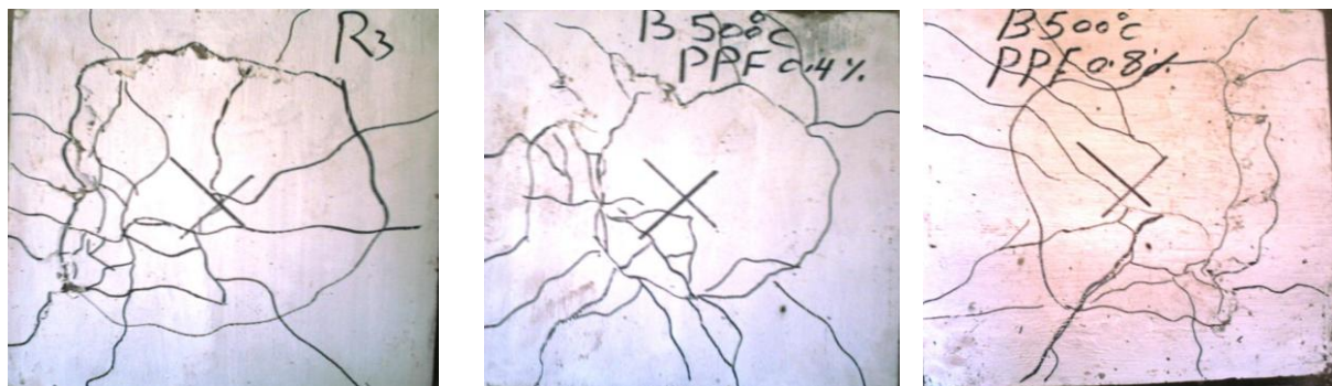
Plate (5) Failure mode for G3 slabs
