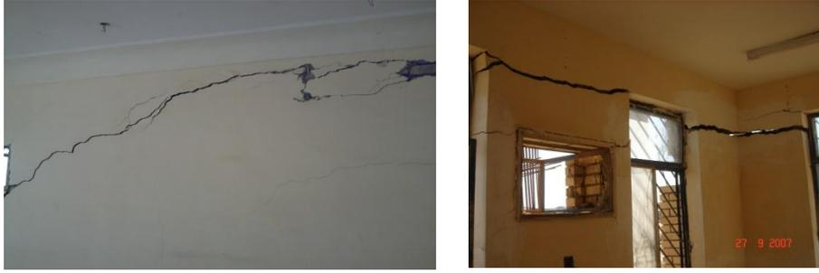
Fig (3) shows the cracks because the settlement
