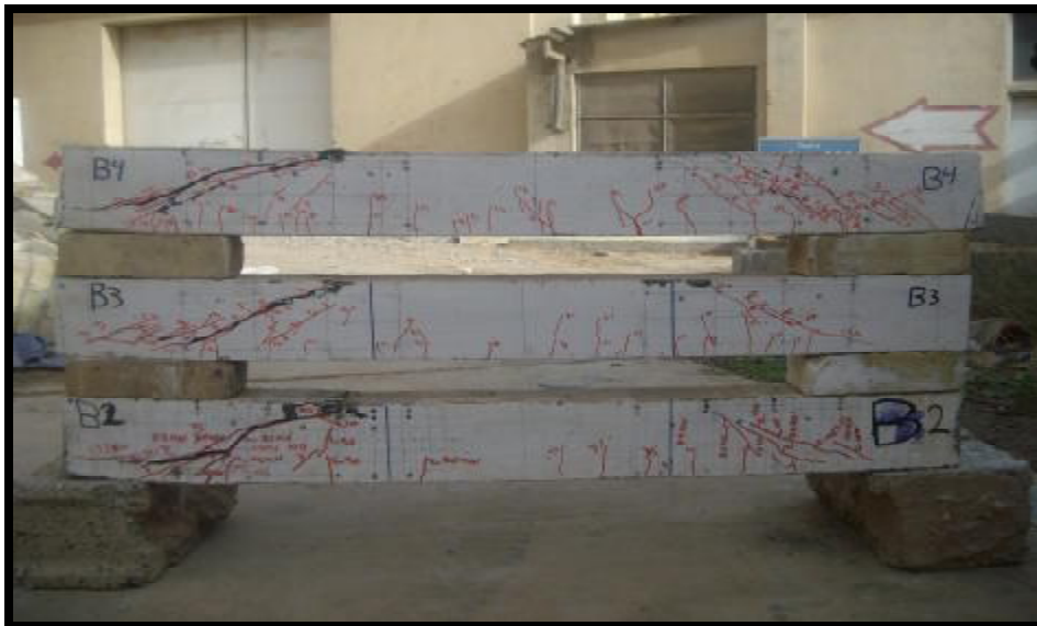
Figure (4): Crack Patterns for Fibrous Beams B2, B3 and B4.
