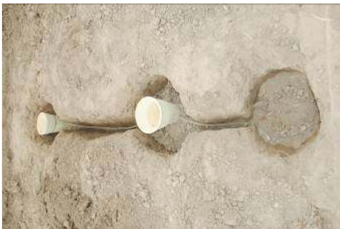
c- Fixing the water supply pipe tightly.
