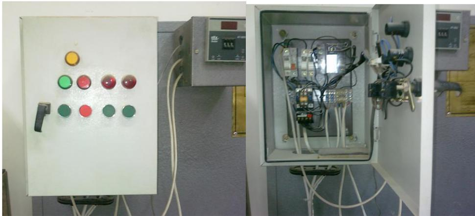
**Figure (9) the Controller Unit of the Solenoid Directional Valve.**
